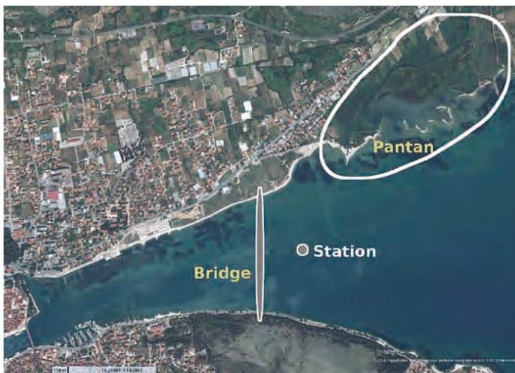
Fig. 1 - Location of bridge, Pantan area and measuring.
